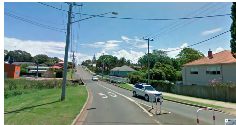
View west along Hill Street at Lord Street showing Wrights Creek corridor and timber pedestrian bridge
