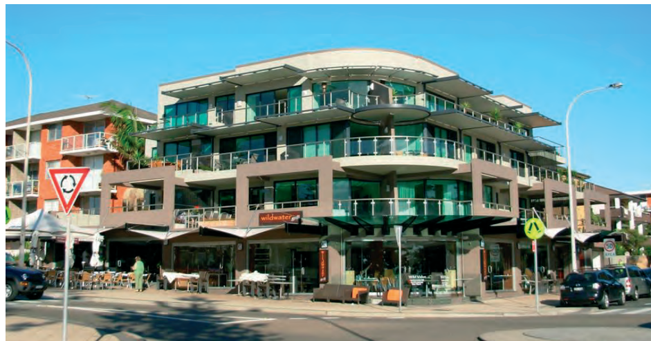
High-density shop-top housing with taller built form; Dee Why NSW
