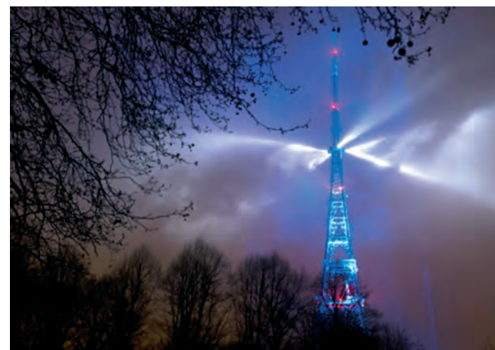
Night lit local telecommunications tower - a creative wayfinding tool and place-making landmark
